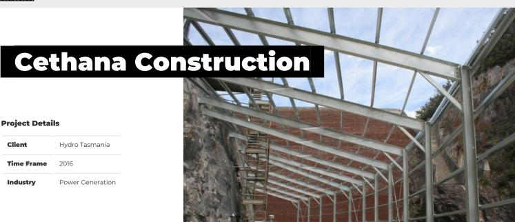
Hydro spray mitigation structure steel work and erection at Cethana Power Station. Architectural Metal Structures Tasmania and across Australia
