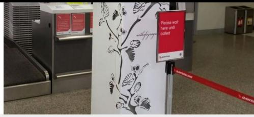
Wrapping of the columns in the check-in area of the Launceston airport in 3mm powder coated steel paneling, laser cut with designs associated with the local area.
