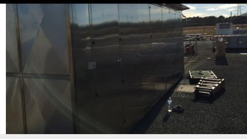
Stainless steel enclosure manufactured for Bell Bay Aluminium to lift up over new switch gear when installed. We offer Steel Fabrication in Sydney, Melbourne & right across Australia
